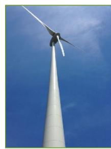
Kaizer Meadow is also the home of a 98 metre tall, 2 MW wind turbine which produces enough electricity for approximately 500 homes. The cost? \$5.5 million!
